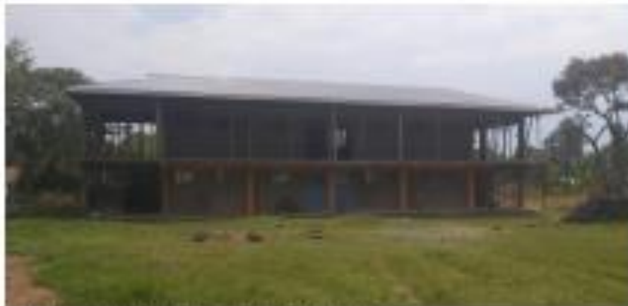
The Bishop Hannington Academy under construction
